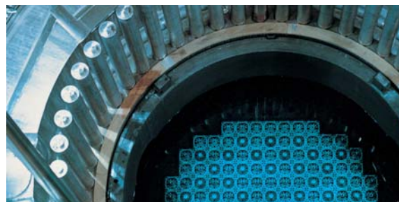
193 fuel assemblies make up the reactor core in which the chain reaction takes place. The open reactor vessel shows the arrangement of the fuel assemblies resembling a chessboard.
