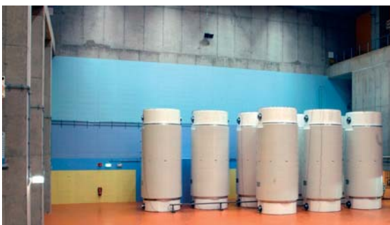
The fuel assemblies are kept in intermediate storage in CASTOR flasks, like here in the on-site interim repository at Lingen, before they are shipped to an ultimate repository.
