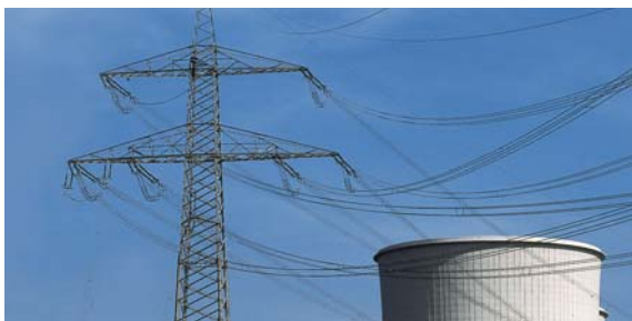
The electricity is transmitted from the Biblis power plant through high-voltage lines to nearby substations from where it is distributed across the interconnected system.
