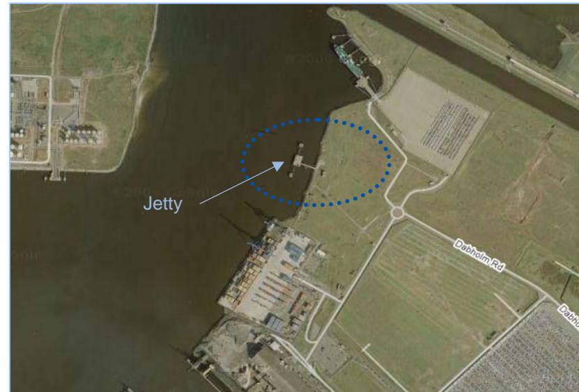
The GasPort Teesside (UK) – Google Earth
