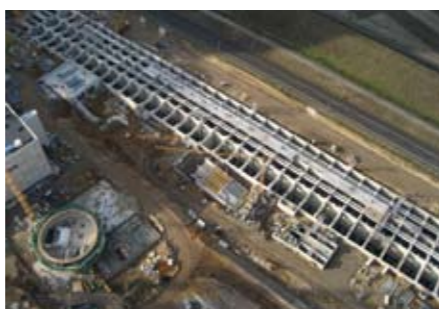
Aerial view of coal bunker, Feb 2008
