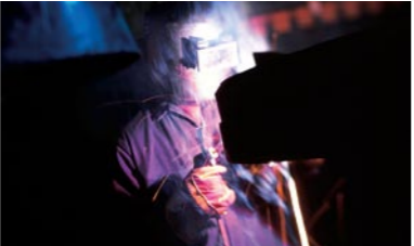
Weld refurbishment at our UK workshop
