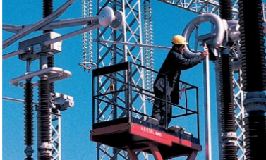
Construction of the 480MW Marmara power station, Turkey
