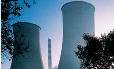
Pego 600MW power station in Portugal commissioned by RWE experts
