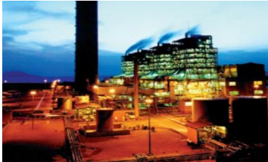
Hub River - 1,292MW oil-fired power station, Pakistan
