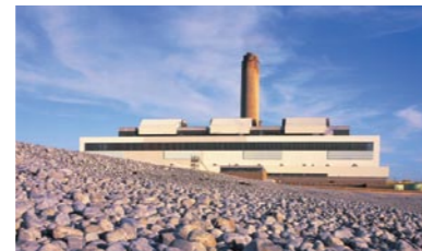
Aberthaw power station
