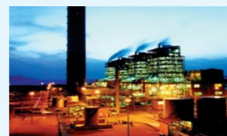
Hub River – 1,300MW oil-fired power station, Pakistan
