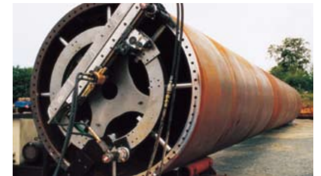
On-site machining of a wind turbine generator tower joint face
