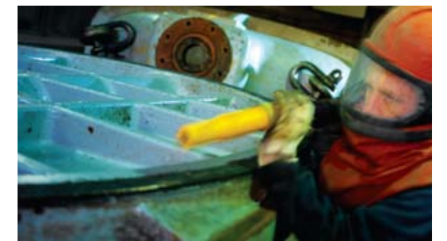
Blast cleaning using latest sponge blast technology
