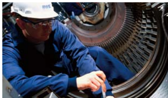
Turbine bearing check
