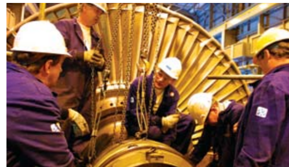
Refurbishment of large LP steam turbine Right: Heavy machine shop
