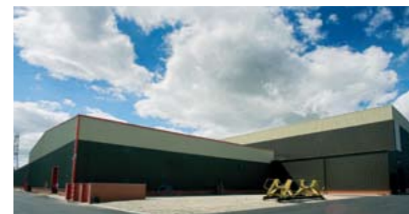
Rotor overhaul building
