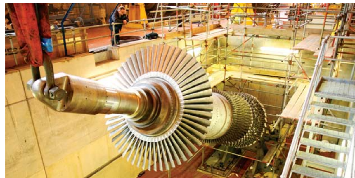
Lowering of a rotor after re-stack
