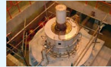
Refurbished Kaplan Unit at Kielder
