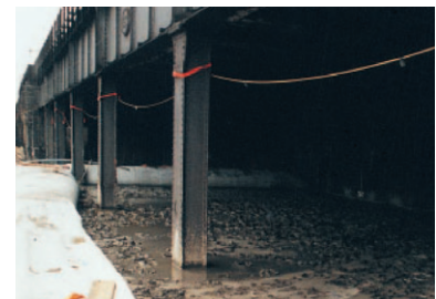
Positioning of first grout bags
