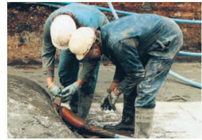
Injection pipe being connected to grout bag
