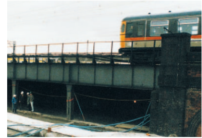
Mass infill shortly after placing
