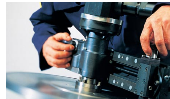
On-site machining of a flange face
