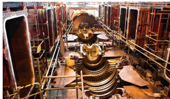
Overhaul of Didcot steam turbine
