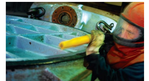
Blast cleaning using latest sponge blast technology
