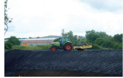
PFA being compacted on built up embankment
