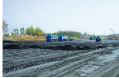
Hauliers and mobile plant on site
