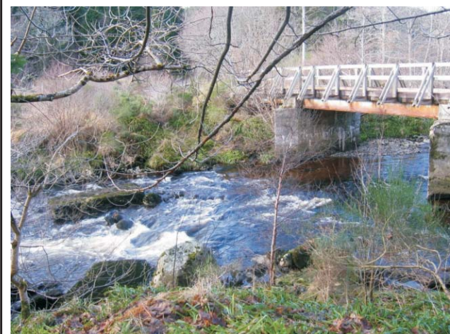
2. Intake location (view from north bank looking south west)
