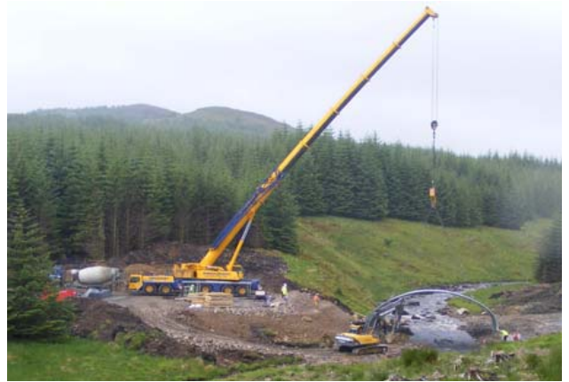
June 2009, Arch being lowered into position.
