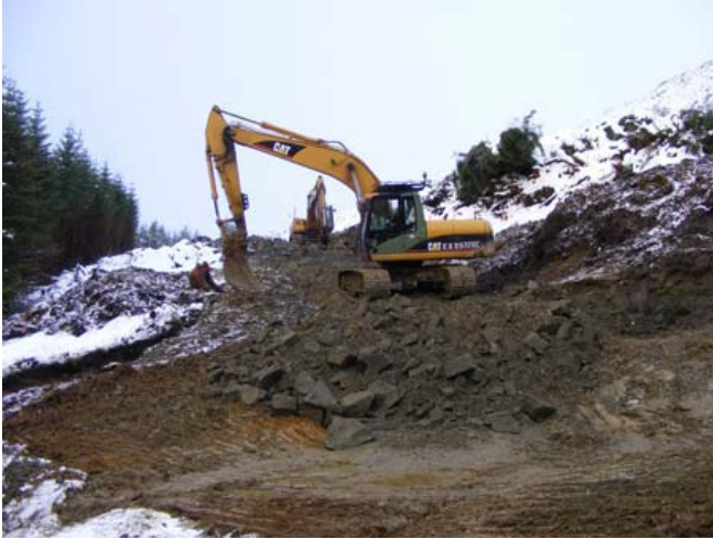
January 2009, Start of western access road.
