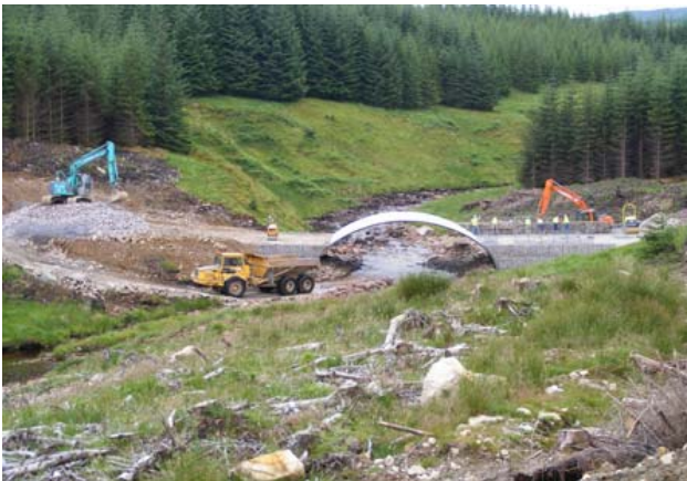
June 2009, Bridge construction.
