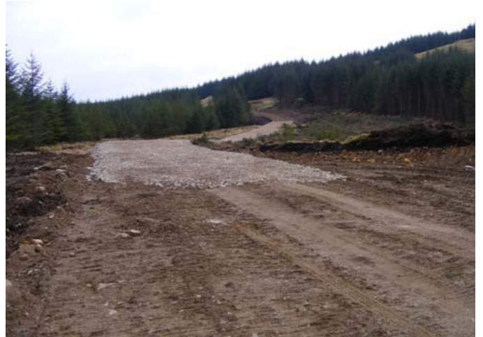
April 2009m Floating road section complete.
