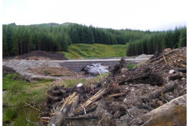
June 2009, Bridge ready for traffic.
