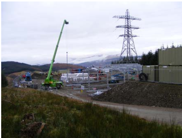
February 2009, Substation construction.
