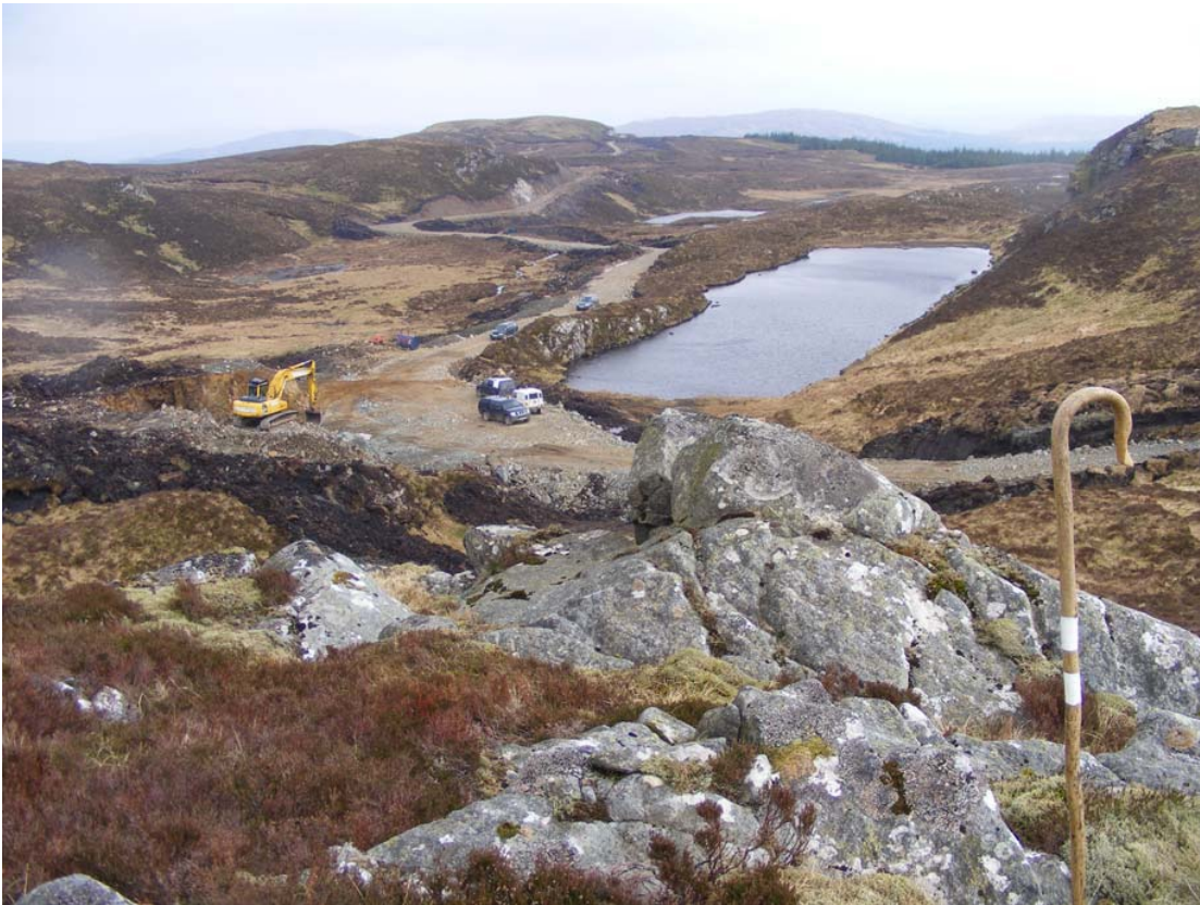
April 2009, Western road to turbine 13.
