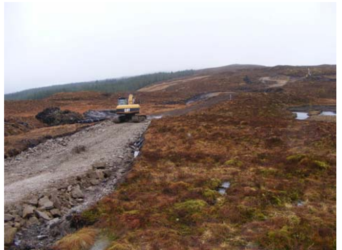
March 2009, Road construction underway.
