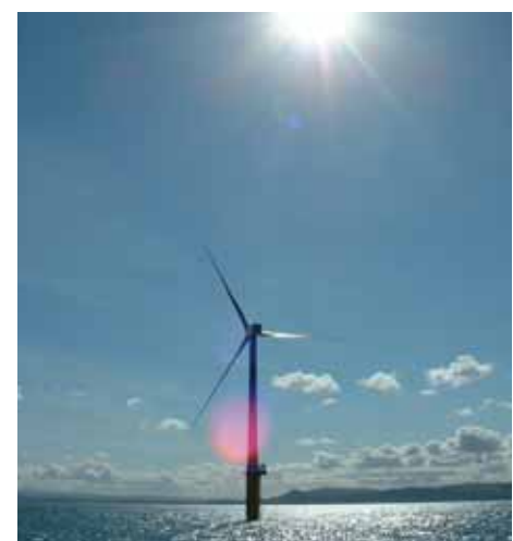
A turbine at North Hoyle Offshore Wind Farm.
