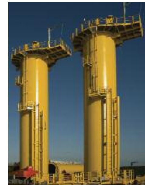
Transition pieces stand erect at Mostyn Dock awaiting transfer to the wind farm site.
