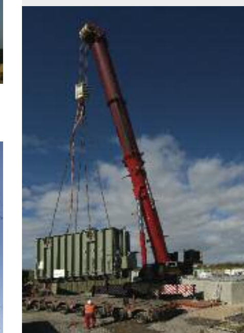
The transformer is delivered to the substation site.
