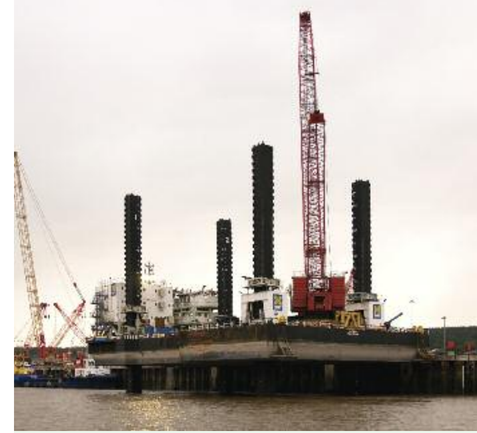
Jack-up barge Lisa in port at Mostyn Dock.
