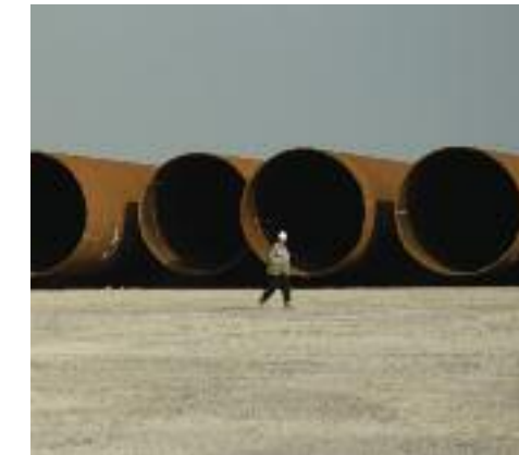
Monopiles laid out at Mostyn Dock.
