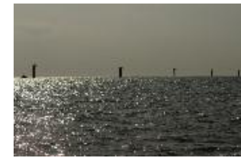
Five completed monopiles and transition pieces.
