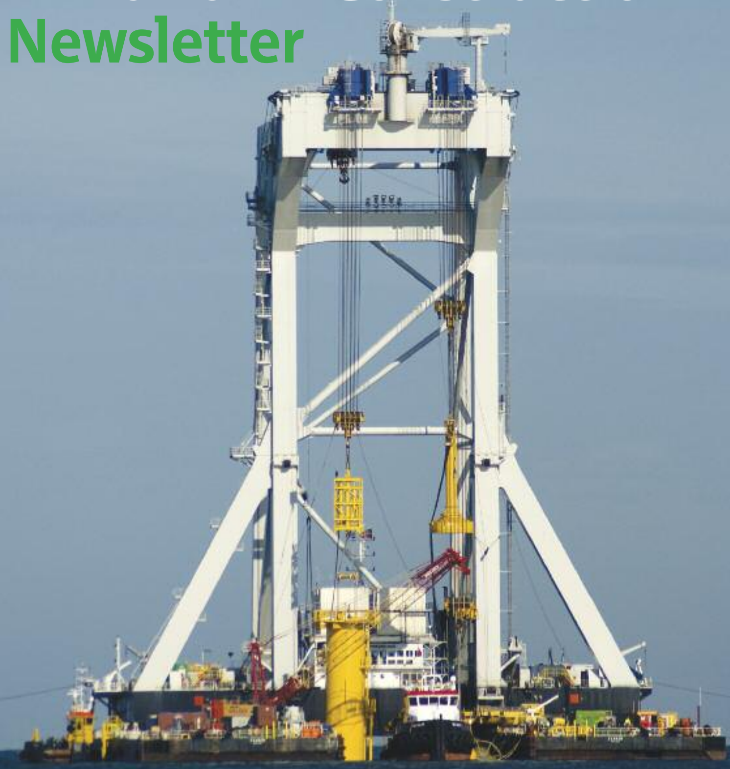
Front cover: A transition piece is fitted over one of the foundation piles at Rhyl Flats Offshore Wind Farm
