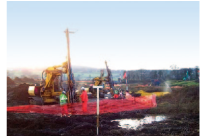
Grouting holes being drilled on site
