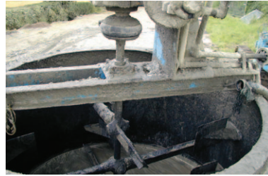
Grout mixture being prepared
