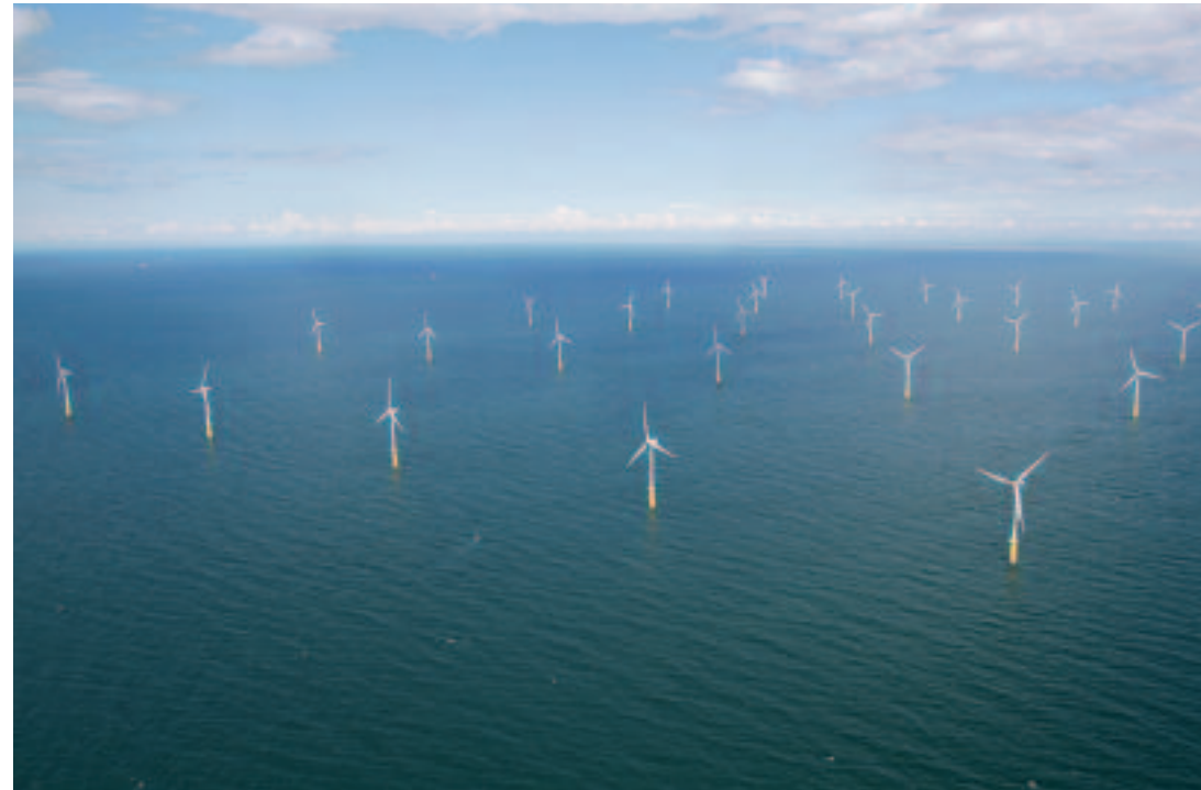
The Operating North Hoyle Offshore Wind Farm.
