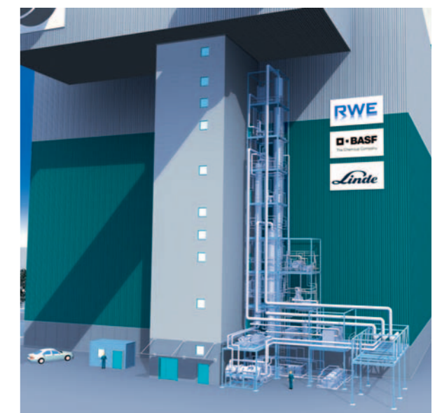
Pilot plant for CO 2 flue-gas scrubbing in the BoA unit at Niederaussem
