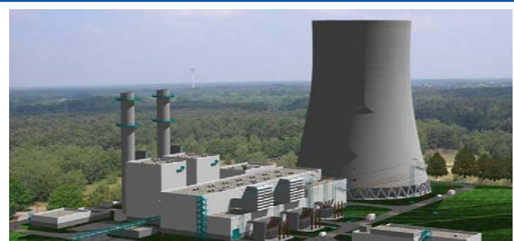
New gas-fired 875 MW plant, > 58% efficiency for peak times
