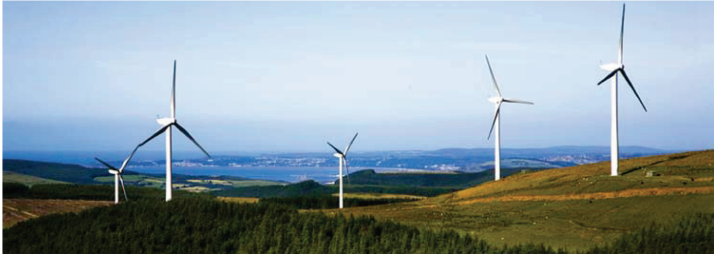
Ffynnon Oer Wind Farm – 2 megawatt turbines, 58 metre tower, 70 metre rotor diameter. (Photographs of existing operational wind farms within this newsletter are not intended to represent the appearance, size or scale of the proposed Brechfa Forest Wind Farms.)
