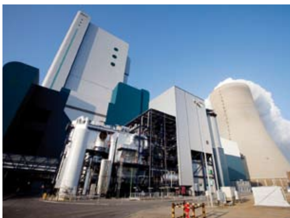
Niederaussem power plant with BoA unit and WTA in the foreground.
