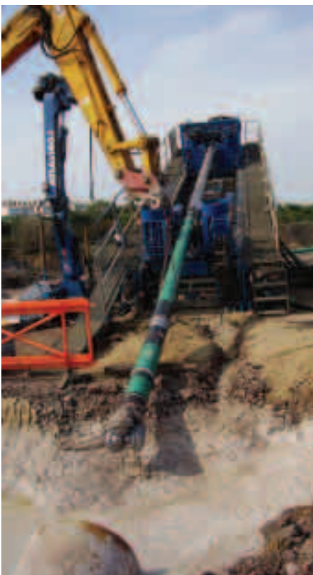
Standard drilling rig
