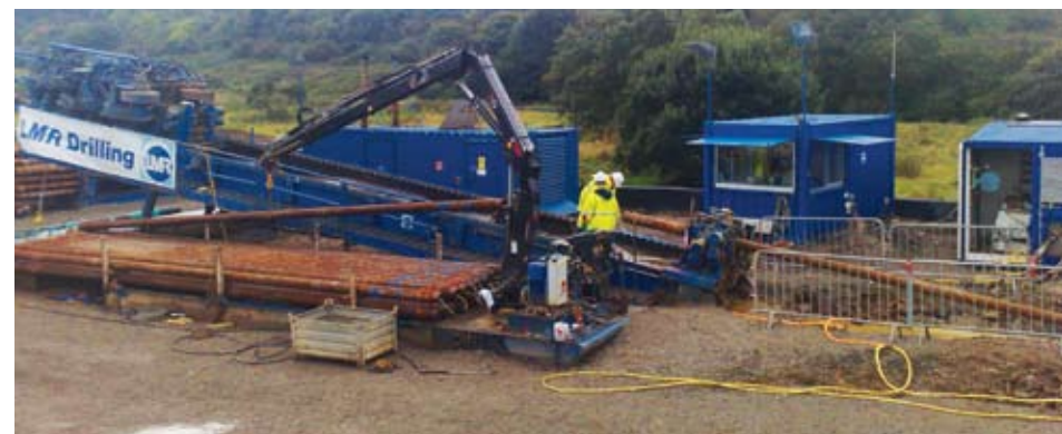
A drilling rig
