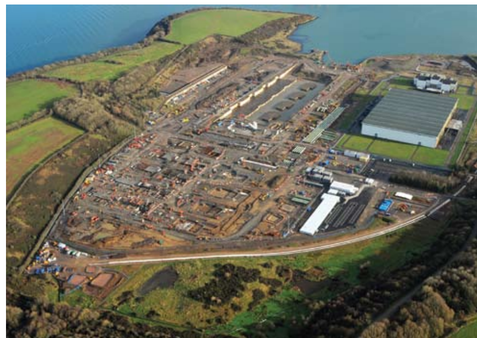
An aerial view of the Pembroke Power Station site
