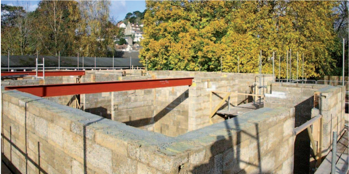
Durisol blocks used during the construction of Branton School, Devon
