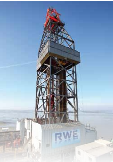
Top: The Drilling and Production Island, viewed from the west.
