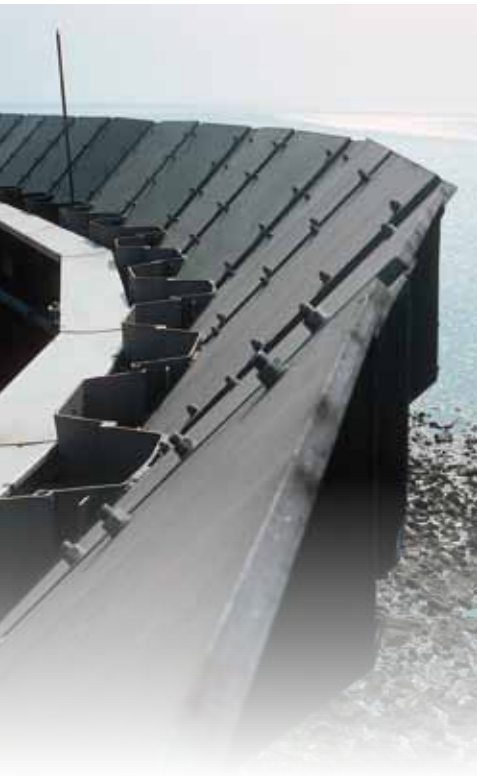
Top: Sheet pile wall with wave deflector. On the sea side, the sheet pile wall extends to a height of 11 metres. Nothing can enter from the outside, apart from rain and spray. And nothing can escape to the outside, not even rain water.
