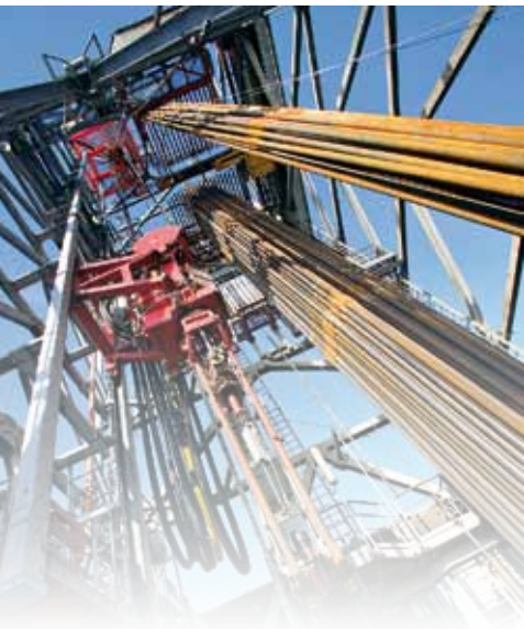
Top: Experienced crews ensure safe drilling operations.
