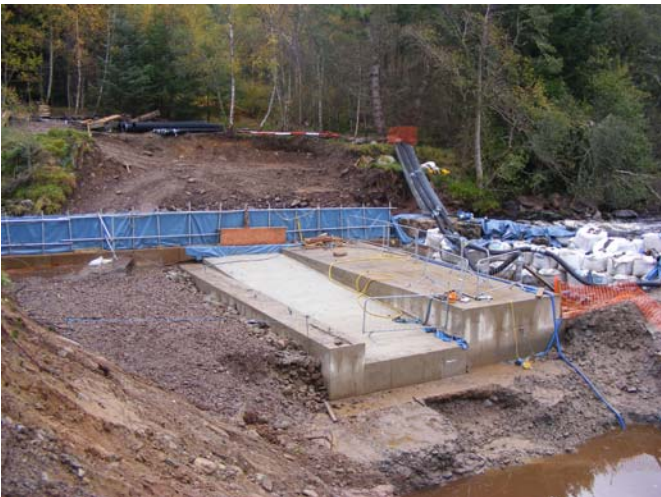
October 2010 – intake base poured
