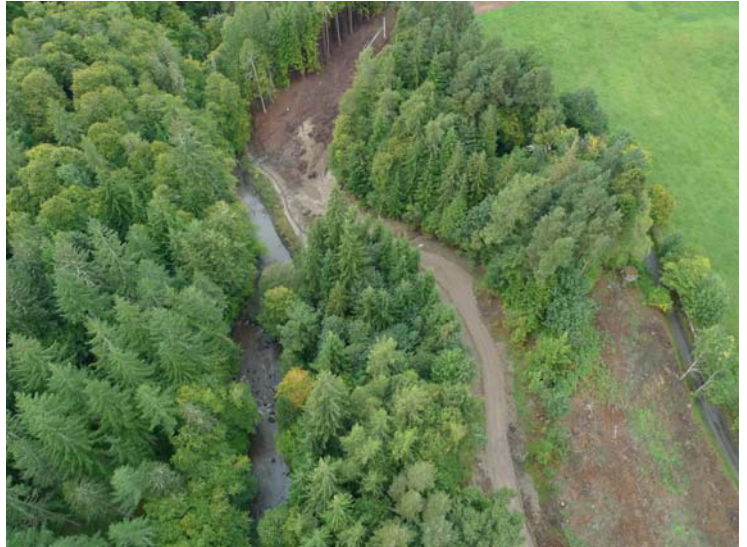
September 2010 – Powerhouse area from above
