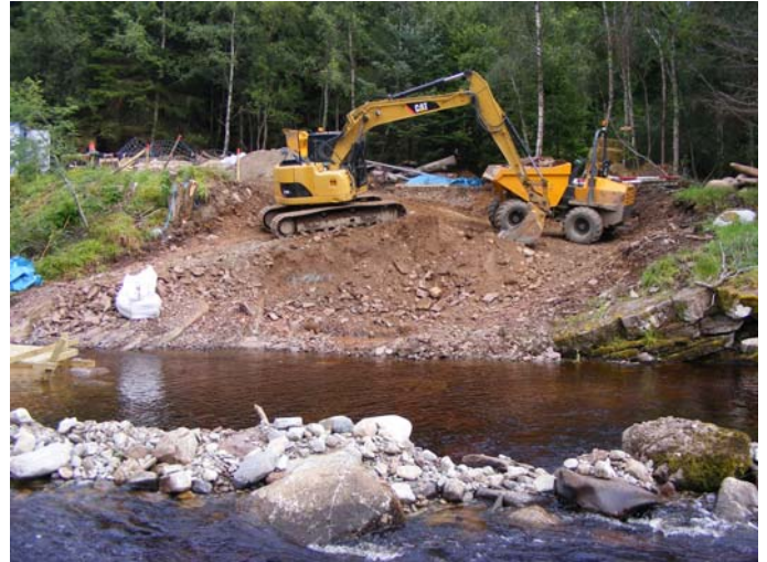
July 2010 – excavation works at the intake
