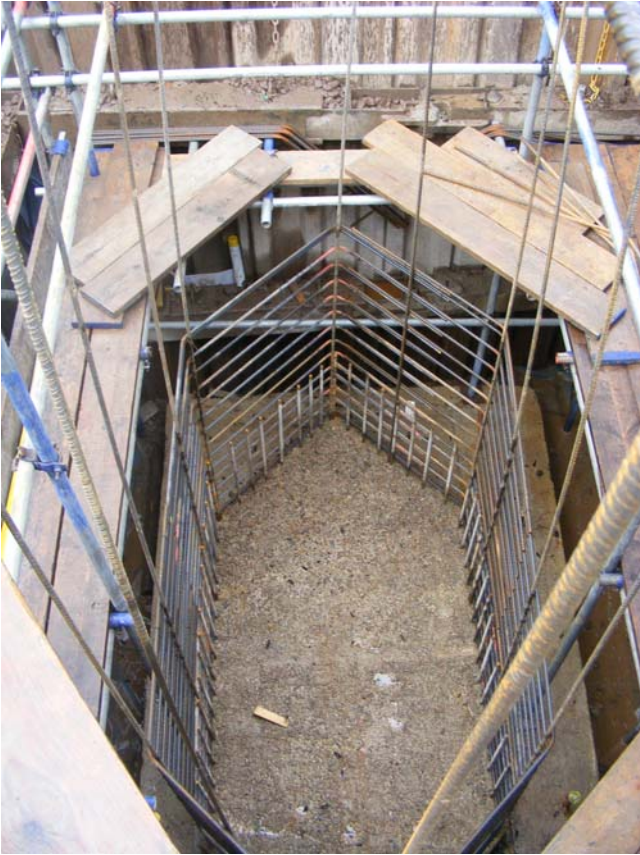
October 2010 – Fixing steel at the north pier
