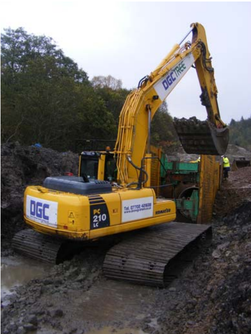
October 2010 – Pipelaying in trench boxes
