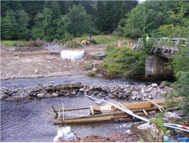
July 2010 – diversion commences at the intake
