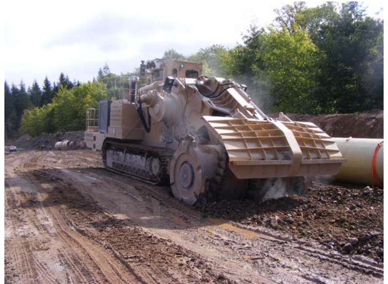
September 2010 – The Rock Hawk in operation in Assynt Fields
