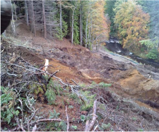
November 2010 – Commencing excavation at powerhouse
