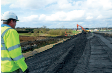
PFA being used as fill to widen the existing M25 embankments
