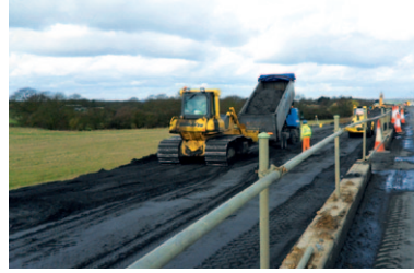
PFA being delivered on site
