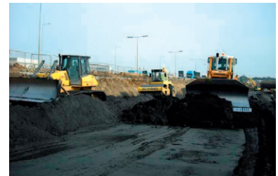
PFA being spread and compacted
