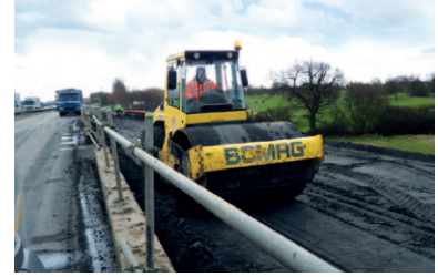
PFA being compacted on site
