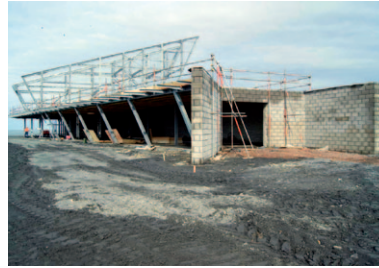
ACE 2 under construction August 2010
