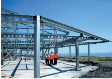
ACE 2 under construction July 2010
