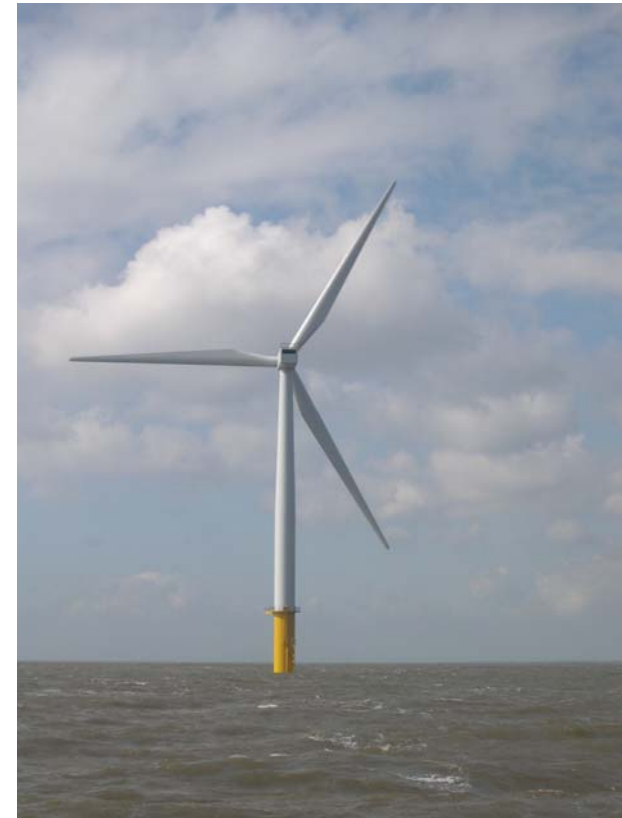
Figure 2: Typical three-bladed offshore wind turbine
