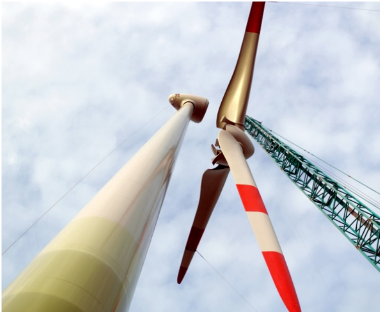
Fig. 1: Dismantling a wind energy converter
