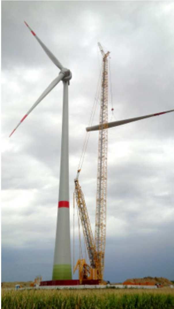
Fig. 3: Rotor blade attached to the crane
