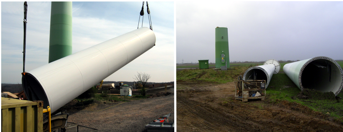
Fig. 16: Steel section when being set down (left), removed steel sections (right)
