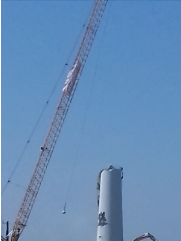
Fig. 14: Demolition by means of an impact weight
