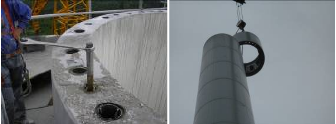
Fig. 10: Re-cutting damaged threads (left); lifting down individual segments (right)
