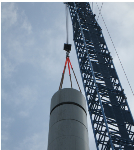
Fig. 11: Attached concrete segment
