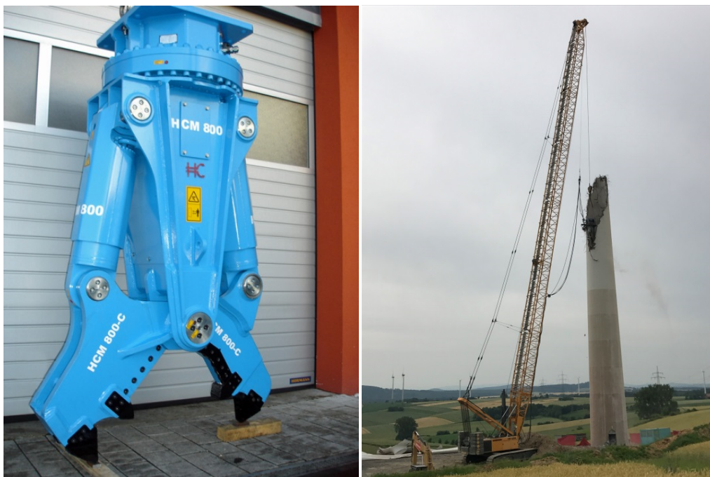
Fig. 12: Demolition excavator with telescopic arm and demolition shears (left); cable excavator (right)
