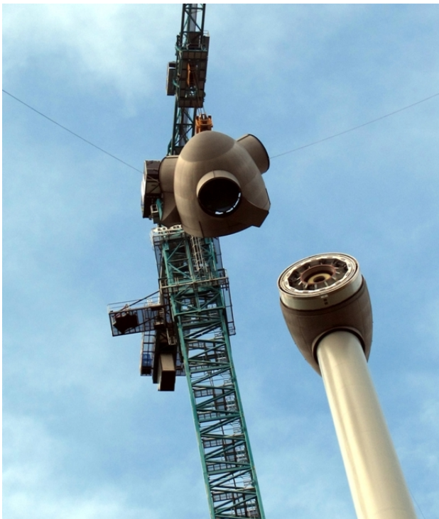
Fig. 4: Rotor head fastened
