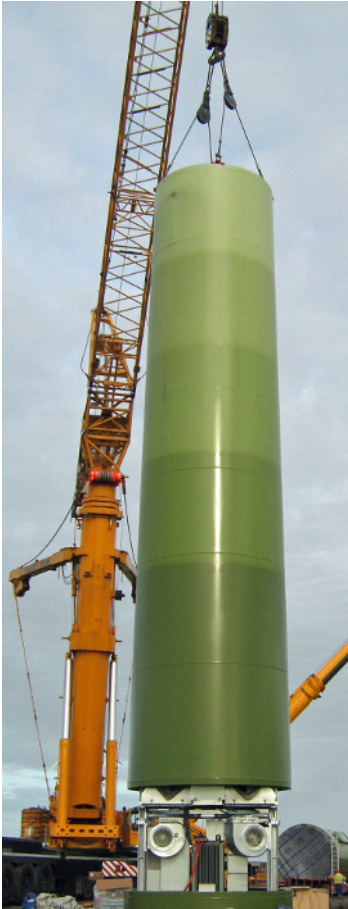
Fig. 6: E-module underneath an attached steel section
