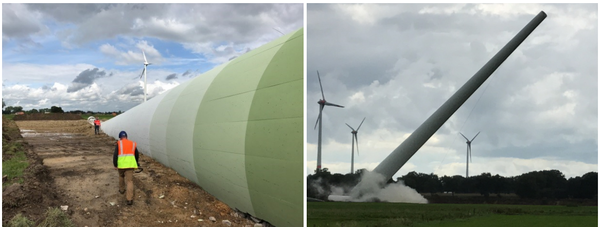
Fig. 13: Brought-down tower (left); controlled felling of the tower (right)
