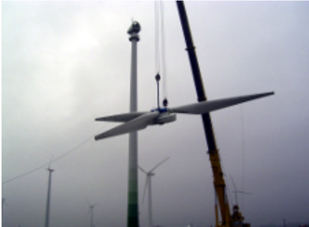
Fig. 2: Lowering the rotor head with rotor blades
