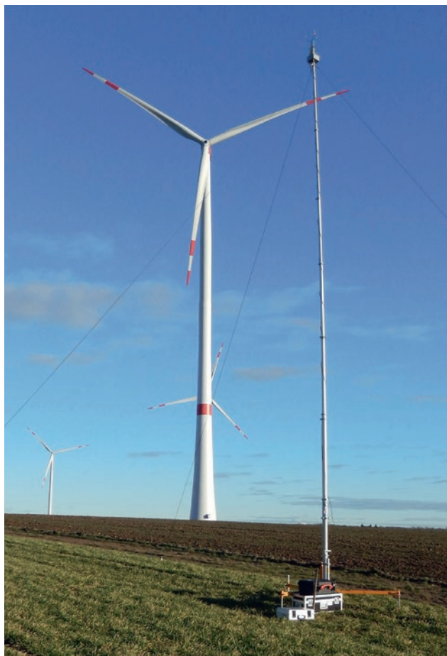
Figure 4.6-1: Wind turbine WT 5 in surroundings used for agricultural purposes. In the foreground you can see the 10 m high wind measurement mast. Photo: Wölfel company
