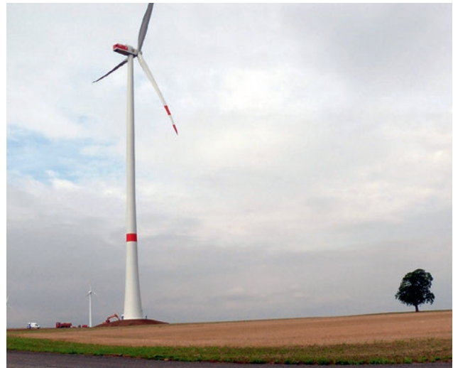
Figure 2-1: Wind turbines – how much infrasound do they emit? Photo: Wölfel company
