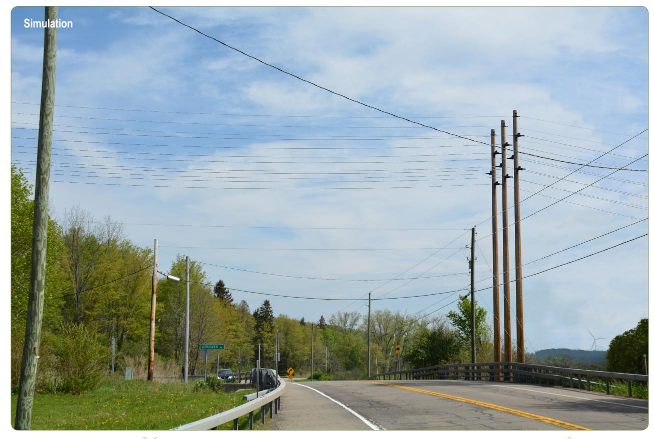
Figure 13: Visual Simulation of Proposed Overhead Collection Line Sheet 2 of 4
