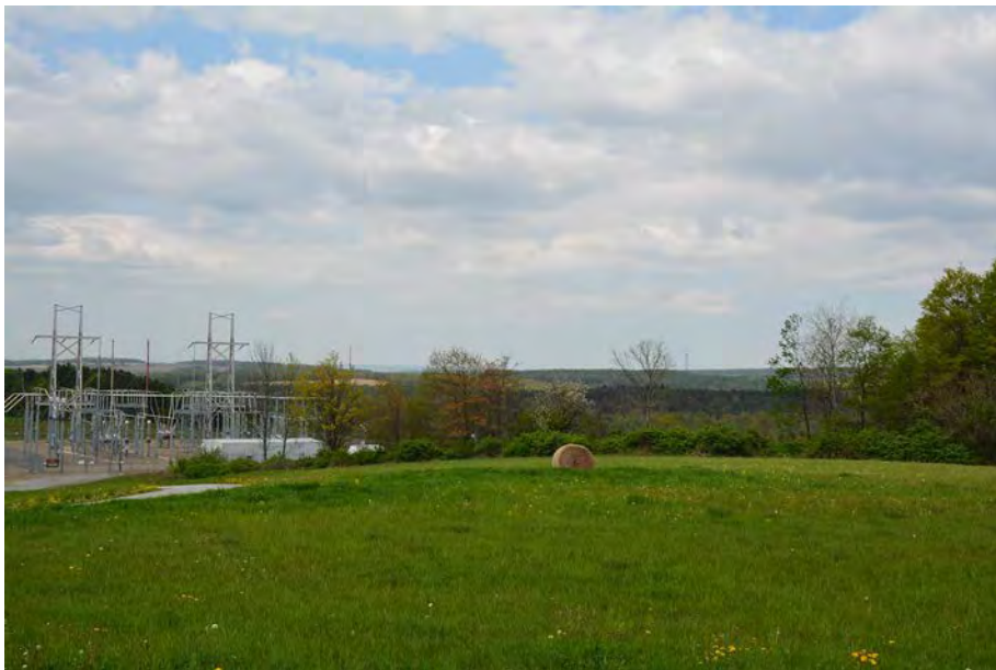
Inset 65: View looking southwest from Van Auker Road at existing NYSEG substation and site of proposed POI substation and collection substation.
