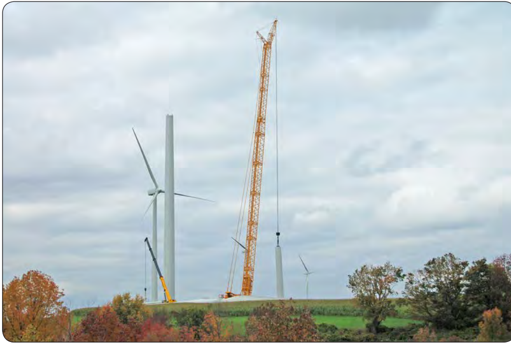
Photo 17 Erection of turbine
