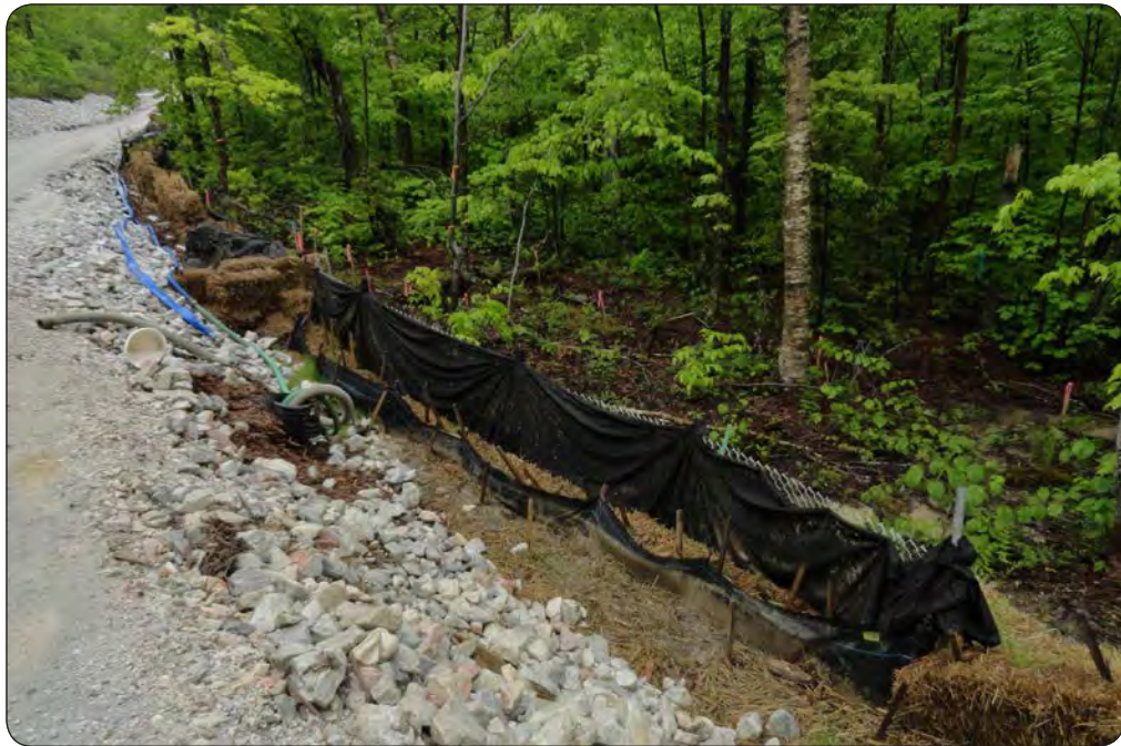
Photo 24 Typical sump pit
