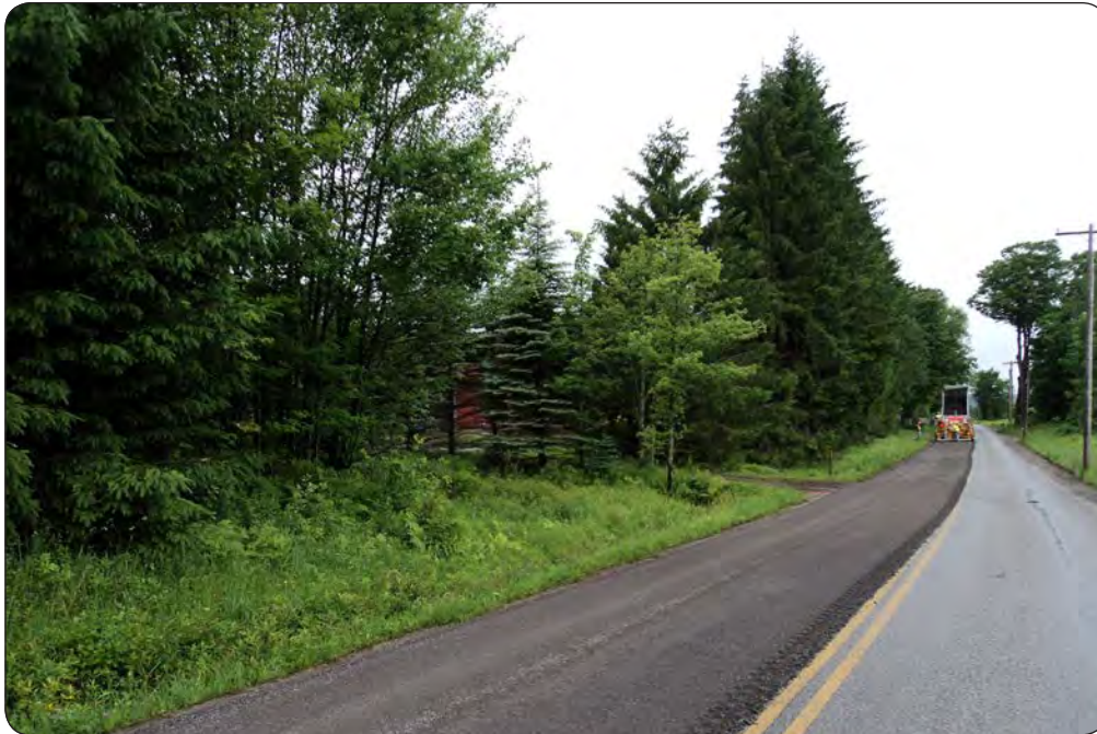
Photo 20 Public road improvement
