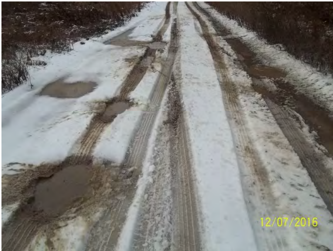
TYPICAL ROAD CONDITION WITH FREQUENT POTHOLES
