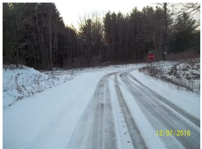
INTERSECTION OF WALTER KURTZ RD AND LANDER RD LOOKING WEST
