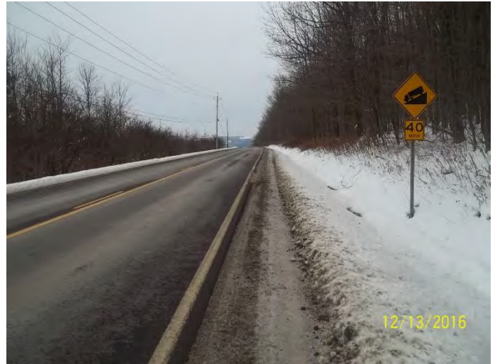
SLOPE WARNINGS BETWEEN REYNOLDS CREEK RD AND EAST LAKE RD
