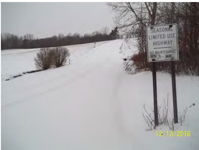
SEASONAL ROAD, NOT PLOWED IN WINTER
