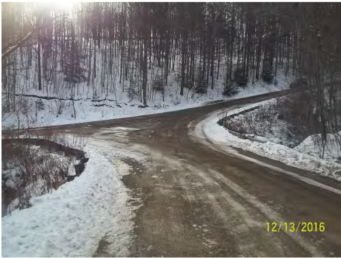
INTERSECTION OF WAGER RD AND GRUBER RD LOOKING SOUTH
