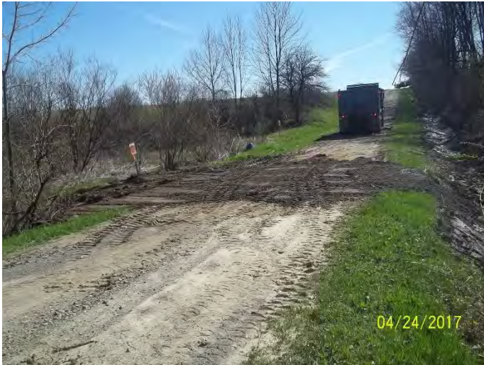
RECENTLY REPLACED IRON CULVERT
