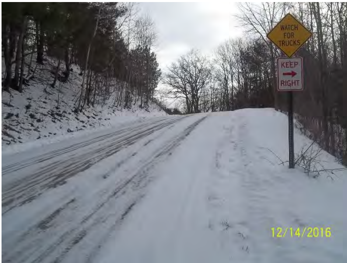
SHARP BLIND CURVES ON STEEP GRADES BETWEEN NY 21 AND CR 92
