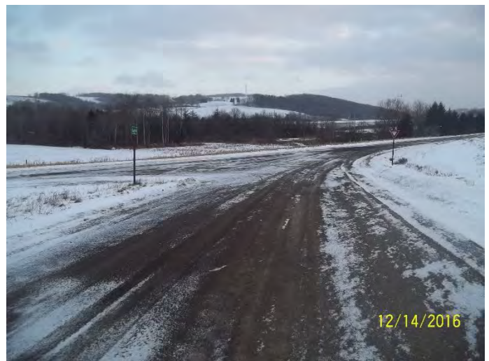
INTERSECTION OF QUANZ RD AND OLD ROUTE 15 LOOKING NORTH
