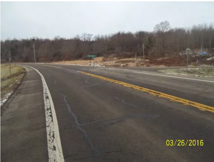
INTERSECTION OF NY 21 AND MACK SCHOOL RD LOOKING WEST
