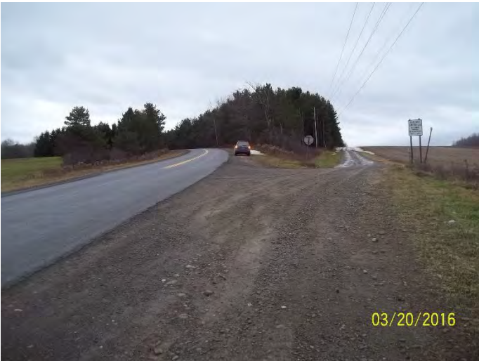
INTERSECTION OF CR 55 AND TUTTLE RD LOOKING SOUTH
