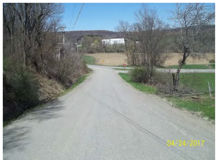
INTERSECTION OF JONES RD AND CR 55 LOOKING NORTH
