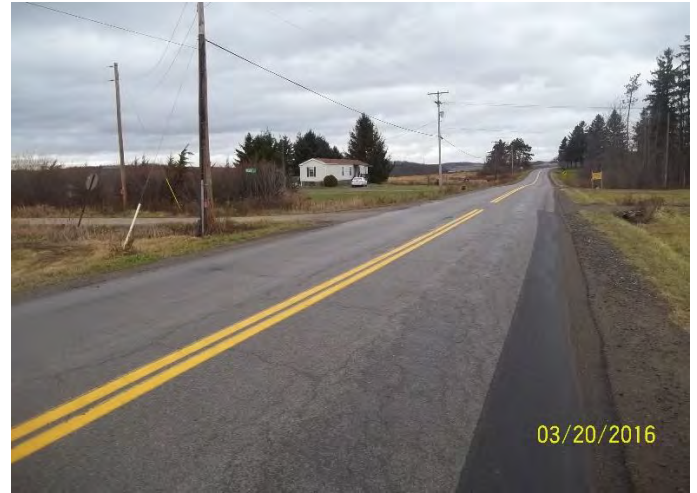
INTERSECTION OF CR 70 AND WELCH RD LOOKING NORTH
