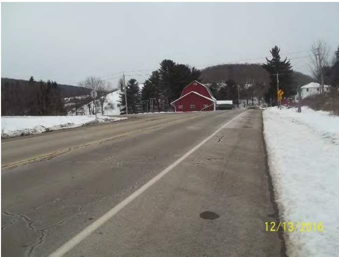
INTERSECTION OF CR 121 AND LAKE HOLLOW RD LOOKING WEST
