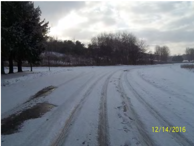
INTERSECTION OF CR 92 AND HENRY DRUM RD LOOKING SOUTH
