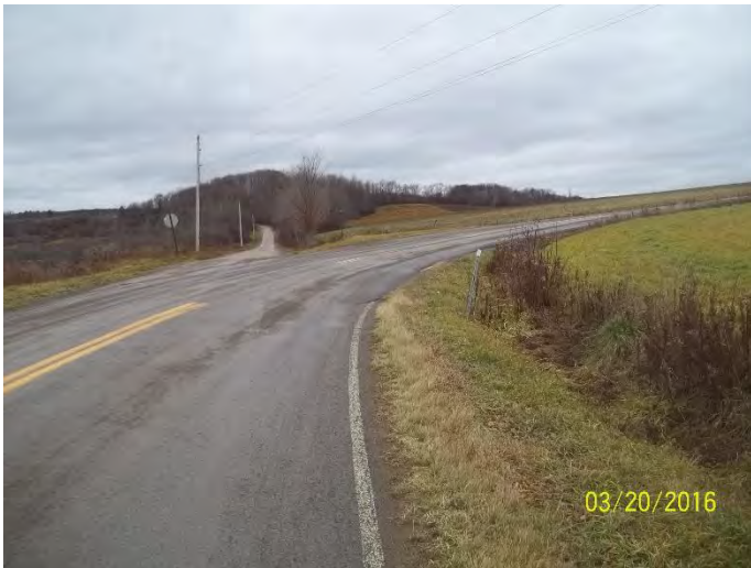
INTERSECTION OF CR 70 AND AVERY LOOKING WEST
