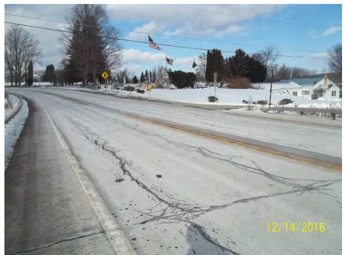
INTERSECTION OF NY 21 AND DAVIS RD LOOKING NORTHEAST
