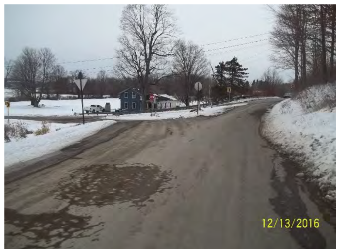
INTERSECTION OF CR 121 AND S CHURCH RD LOOKING NORTH
