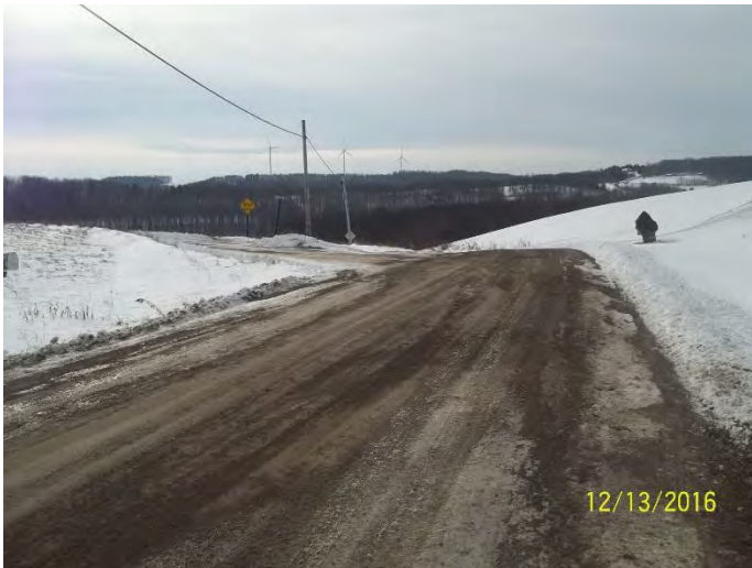
INTERSECTION OF WAGER RD AND WALTERS RD LOOKING SOUTH
