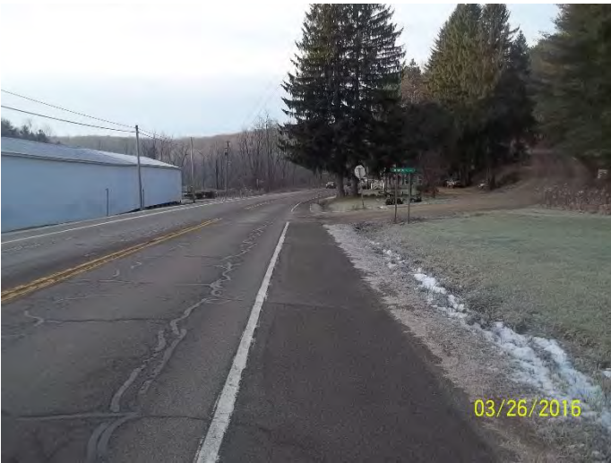
INTERSECTION OF NY 21 AND BABCOCK RD LOOKING SOUTH
