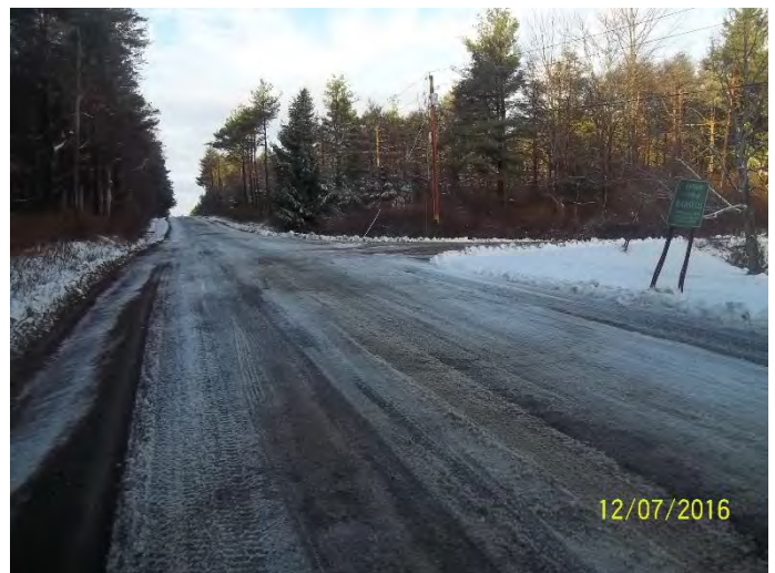
INTERSECTION OF MACK SCHOOL RD AND WAGNER RD LOOKING WEST
