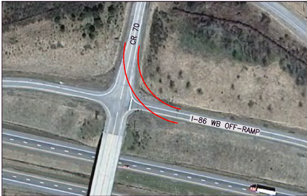
LOCATION 25 - I-86 WESTBOUND OFF-RAMP (EXIT 35) AT CR 70
