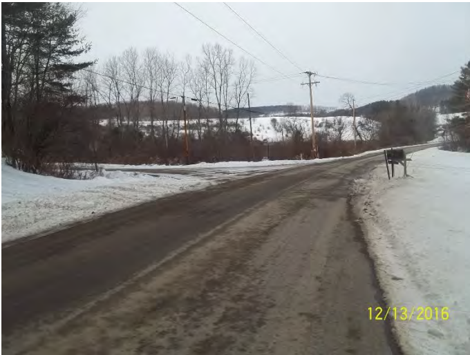
INTERSECTION WITH OILWELL HOLLOW RD LOOKING NORTH
