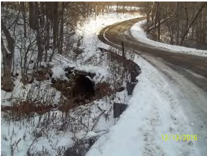
CULVERT AT GRUBER RD INTERSECTION
