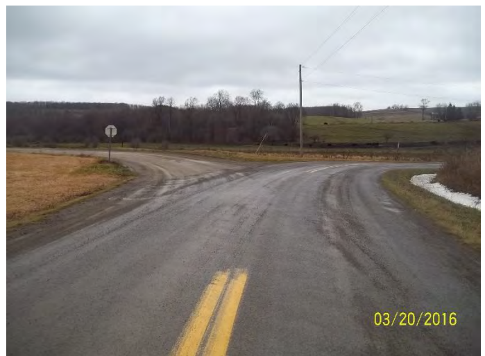
INTERSECTION OF CR 70 AND SAXTON RD LOOKING NORTH
