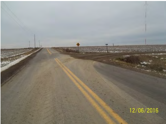
INTERSECTION OF CR 54 AND ROSE RD LOOKING EAST
