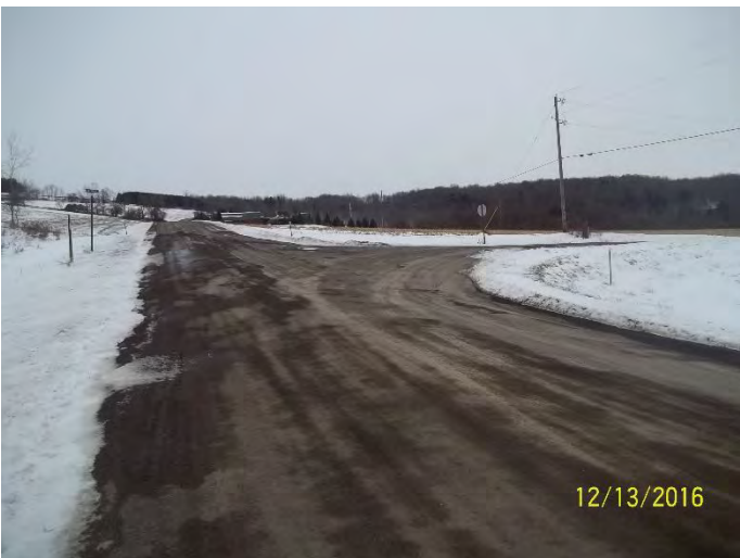
INTERSECTION OF DYE RD AND NEW GALEN RD LOOKING EAST
