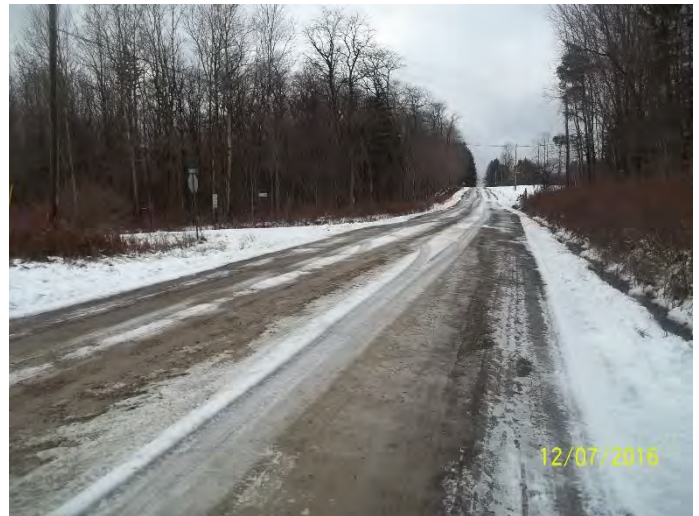
INTERSECTION OF STONE HILL RD AND WAGNER RD LOOKING WEST
