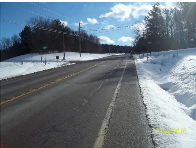
INTERSECTION OF NY 21 AND EMO RD LOOKING SOUTH
