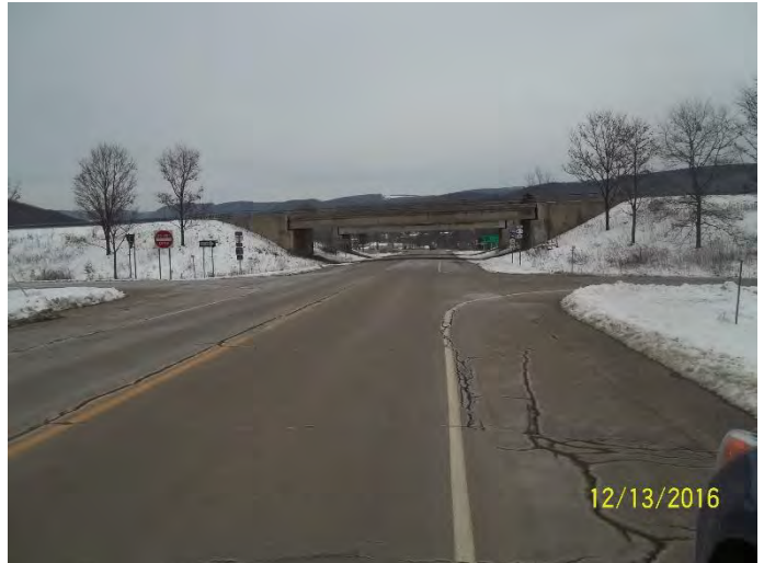
CR 121 AT I-390 LOOKING EAST
