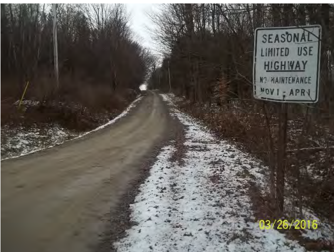
SEASONAL ROAD SOUTH OF CANFIELD RD NOT PLOWED IN WINTER
