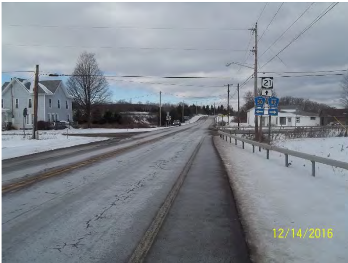
INTERSECTION OF NY 21, CR 92, AND CR 50 LOOKING SOUTH
