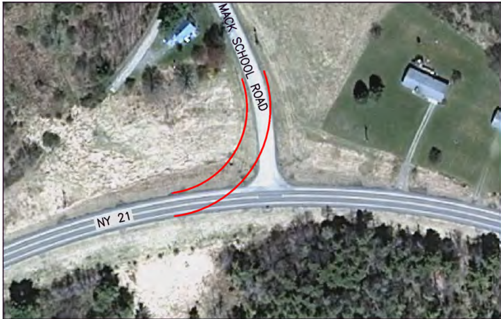
LOCATION 13 – MACK SCHOOL RD AT STATE ROUTE 21
