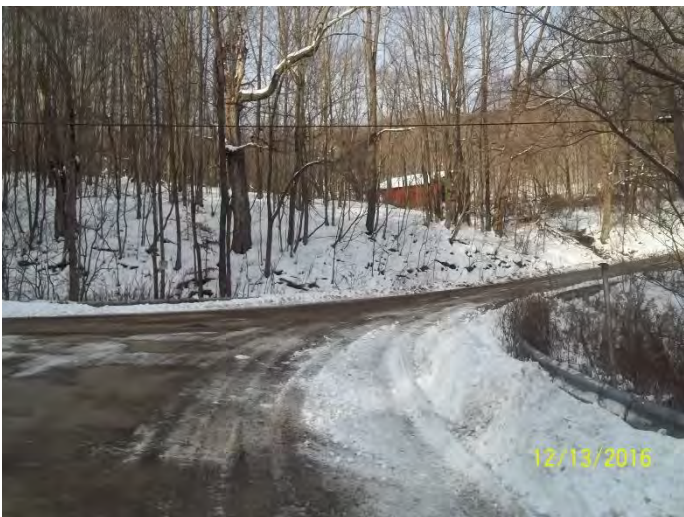
LOW WIRES AT GRUBER RD INTERSECTION
