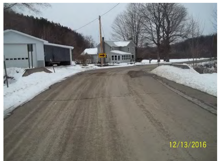
SHARP CURVE OVER CULVERT WITH CONCRETE RAILING NEAR NY 21
