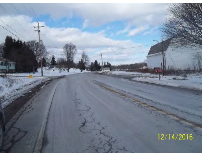
INTERSECTION OF NY 21 AND CR 121 LOOKING NORTH
