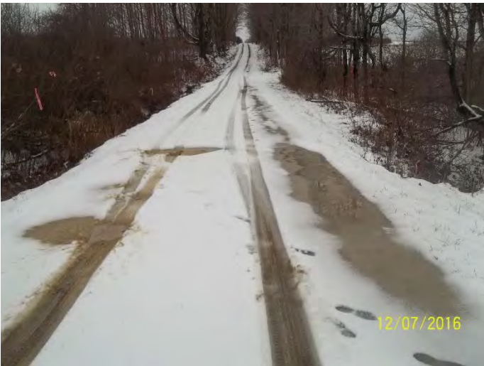
NARROW SEGMENT OVER CULVERT JUST EAST OF DANVILLE/FREMONT TOWN LINE
