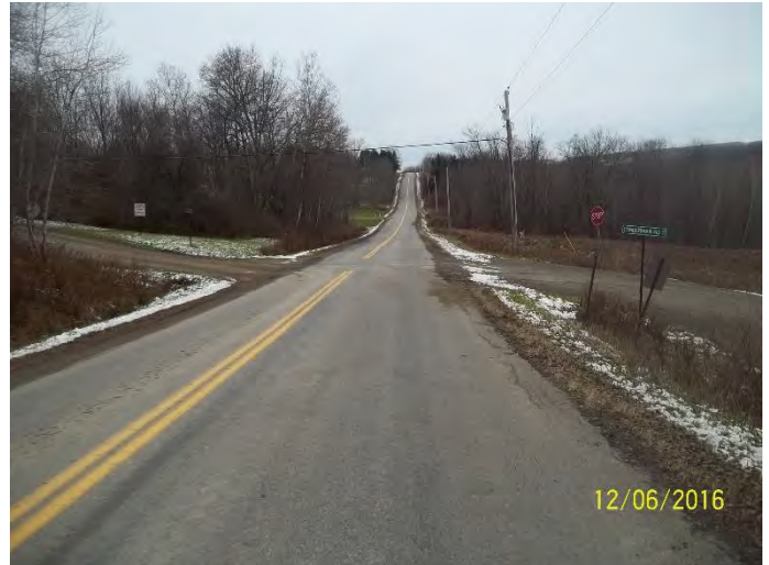
INTERSECTION OF CR 54 AND CONDERMAN LOOKING WEST
