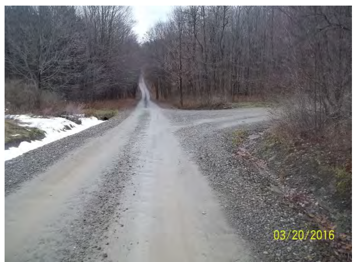
INTERSECTION OF AVERY RD AND STEWART RD LOOKING EAST
