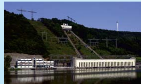
Herdecke pumped-storage power plant
